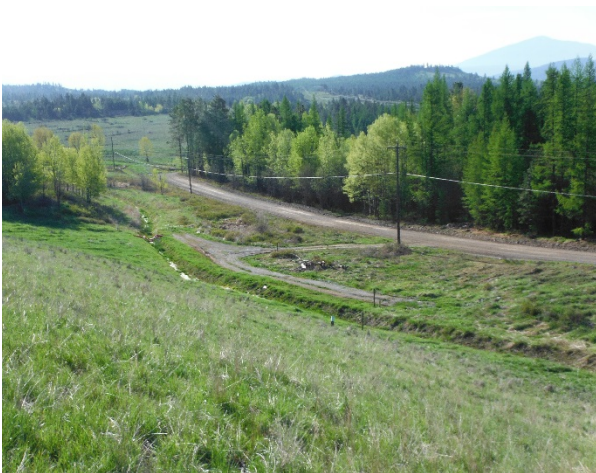
6.05: May 10, 2017 Downstream slope of ARD South Dike
