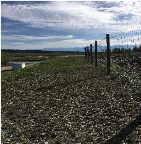
6.21: May 10, 2017 Crest of North Dike
