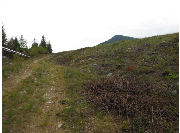
8.02: May 11, 2017 North Dike access ramp
