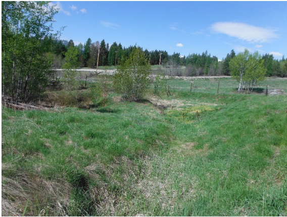
5.03: May 10, 2017 Drainage channel from West Gypsum Dike toe
