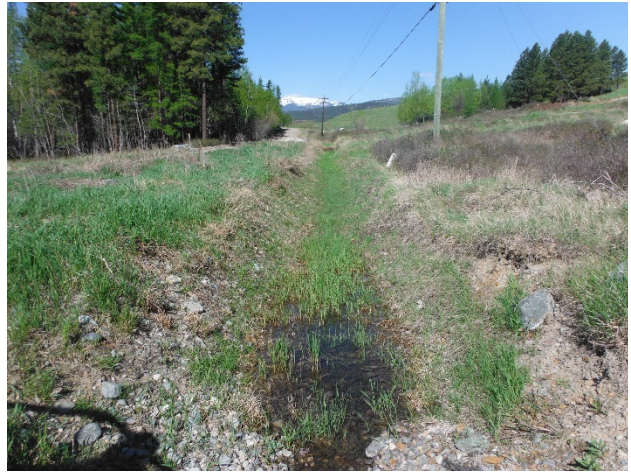
6.10: May 10, 2017 Ditch downstream of ARD Weir #2
