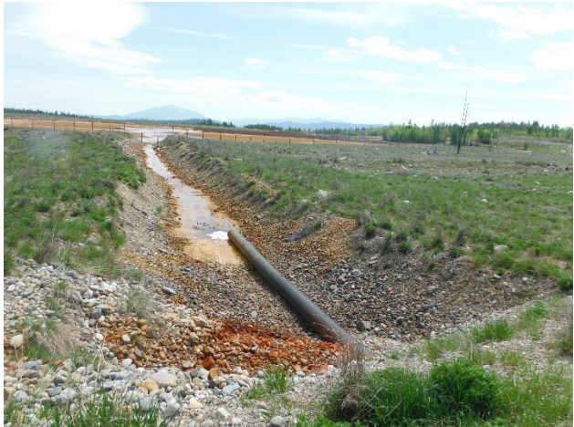
2.03: May 10, 2017 Seepage collection channel from Old Iron Pond
