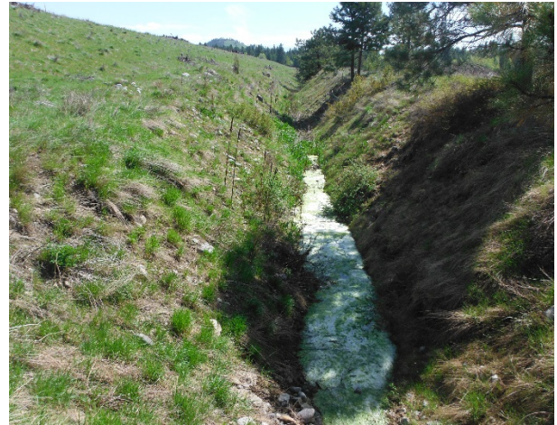
5.16: May 10, 2017 Ditch at toe of East Gypsum Dike
