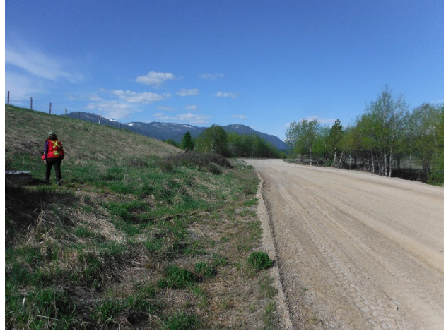
6.14: May 10, 2017 Downstream slope of North Dike
