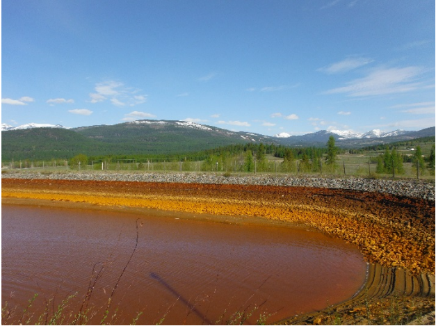
6.13: May 10, 2017 Upstream slope of North Dike
