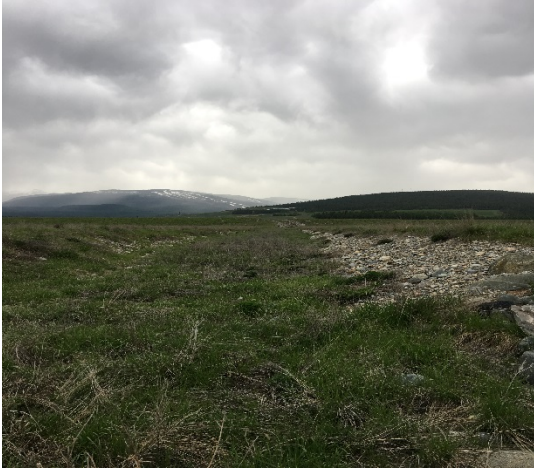
4.13: May 11, 2017 Drainage channel from Dike #1 to Emergency Spillway.
