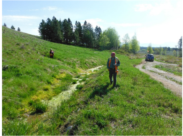
6.08: May 10, 2017 Ditch at downstream toe of South Dike
