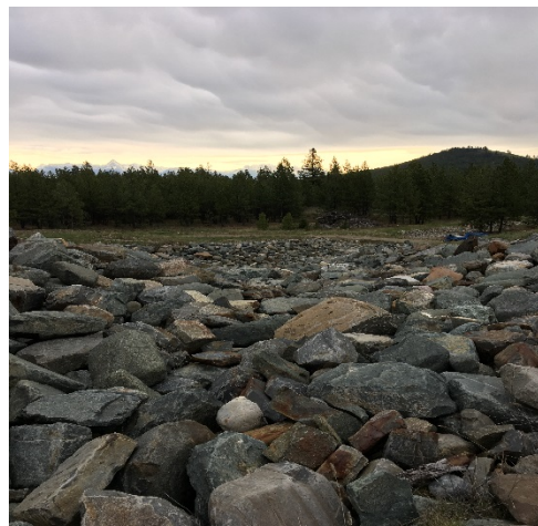
4.12: May 11, 2017 Emergency Spillway
