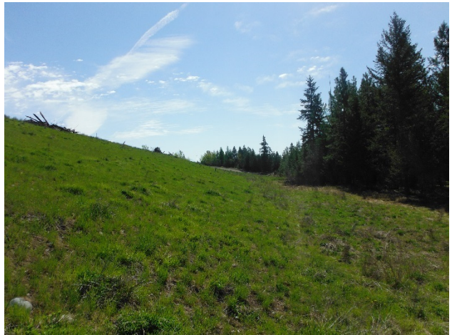
5.06: May 10, 2017 James Creek collects seepage from toe of Gypsum dike
