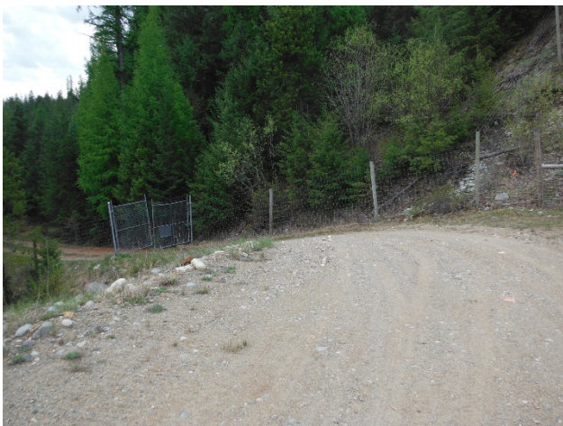
8.11: May 11, 2017 South end access road of South Dike
