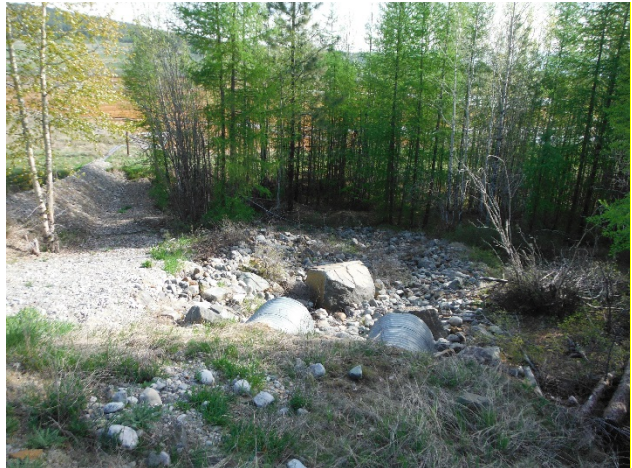
2.04: May 10, 2017 Culverts from ARD Spillway into Emergency Storage Pond
