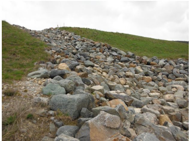
4.10: May 11, 2017 Emergency Spillway
