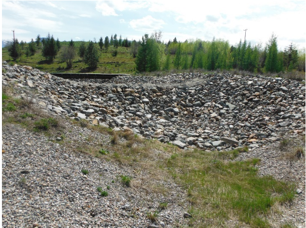
9.01: May 10, 2017 Spillway crest
