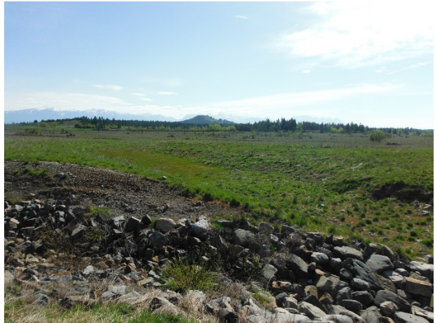
9.04: May 10, 2017 West Gypsum Emergency Spillway
