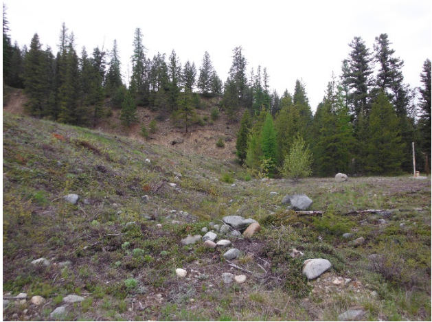
8.01: May 11, 2017 Downstream slope of North Dike
