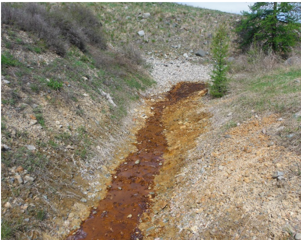
1.17: May 10, 2017 Seepage from toe of Iron Dike.
