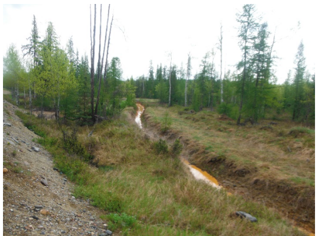
4.06: May 11, 2017 Ditch at toe of Siliceous Pond #2
