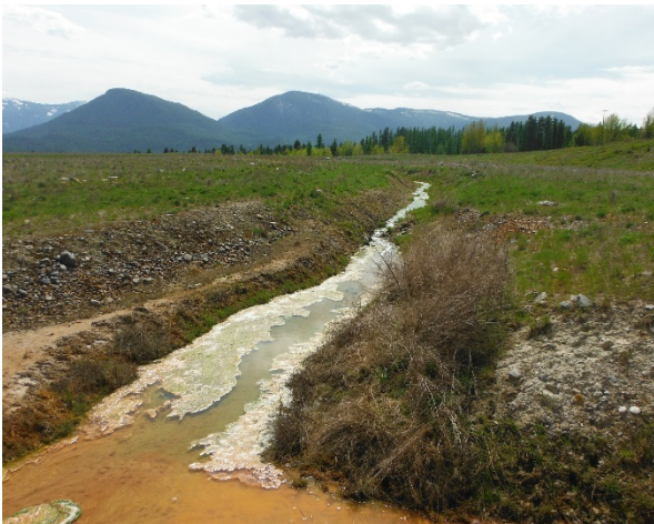
1.15: May 10, 2017 Seepage collection ditch.
