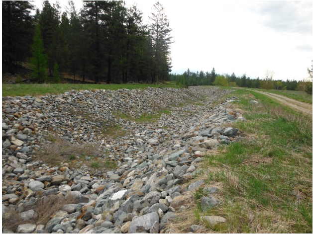
4.01: May 11, 2017 North surface water diversion channel
