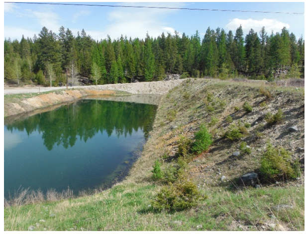
5.34: May 10, 2017 Northeast Gypsum Dike
