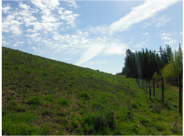
5.02: May 10, 2017 West Gypsum Dike Toe
