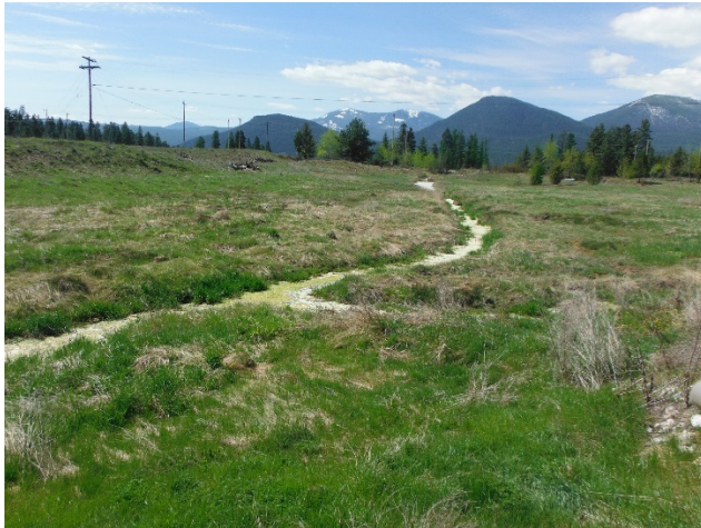
5.15: May 10, 2017 Ditch at toe of East Gypsum Dike
