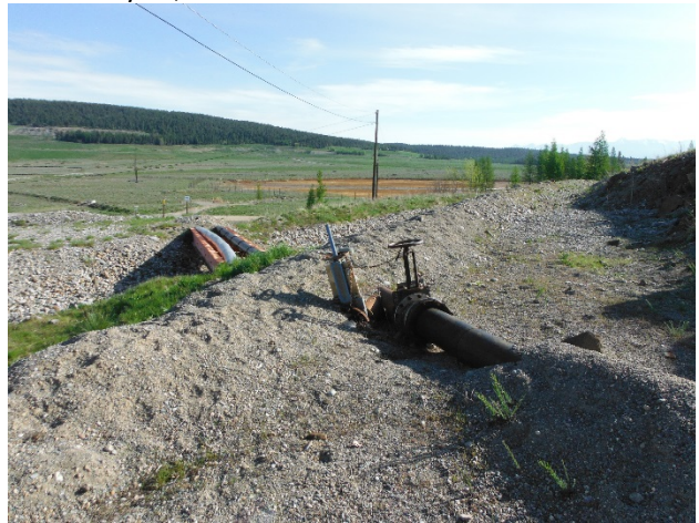
6.12: May 10, 2017 ARD Emergency Spillway
