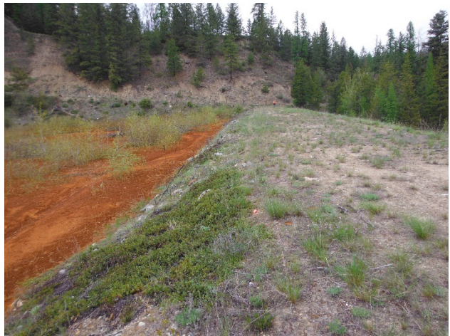
8.04: May 11, 2017 Upstream slope of North Dike
