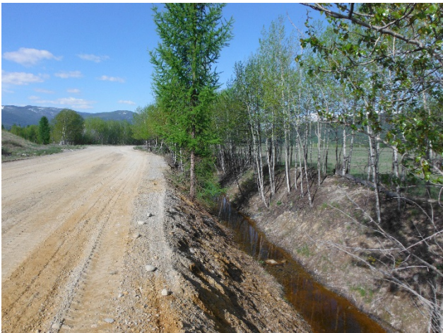
6.15: May 10, 2017 Drainage ditch downstream of North Dike toe.
