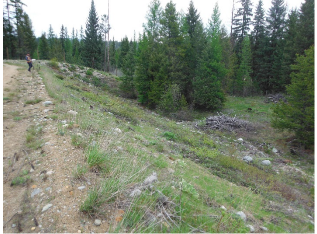
8.08: May 11, 2017 Downstream slope of South Dike
