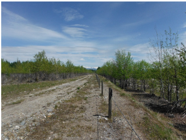
7.03 May 10, 2017 Calcine Pond Dike
