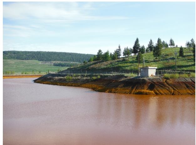
6.30: May 10, 2017 ARD Pond and DWTP Pump Station
