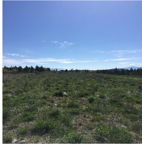
5.08: May 10, 2017 West Gypsum Dike crest
