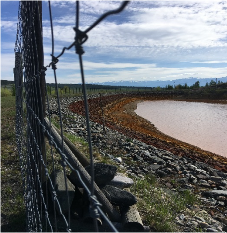
6.25: May 10, 2017 Upstream slope of North Dike
