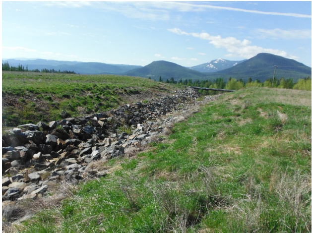
9.03: May 10, 2017 Spillway channel
