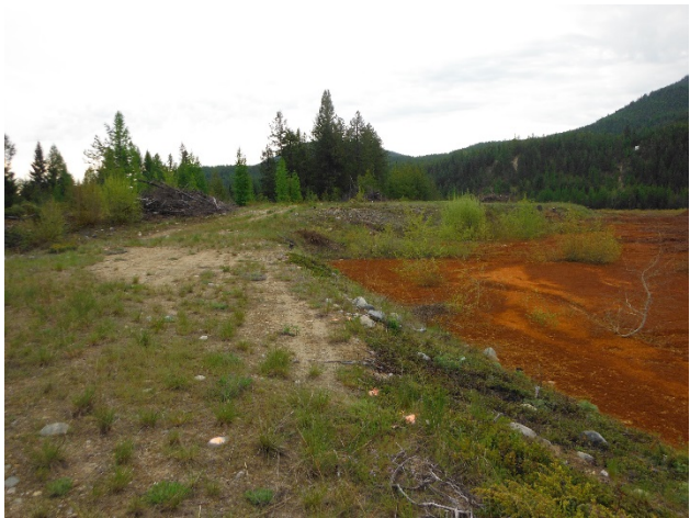
8.03: May 11, 2017 Crest of North Dike
