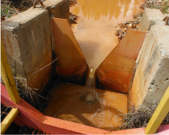
1.13: May 10, 2017 Weir #4 (Old Weir)
