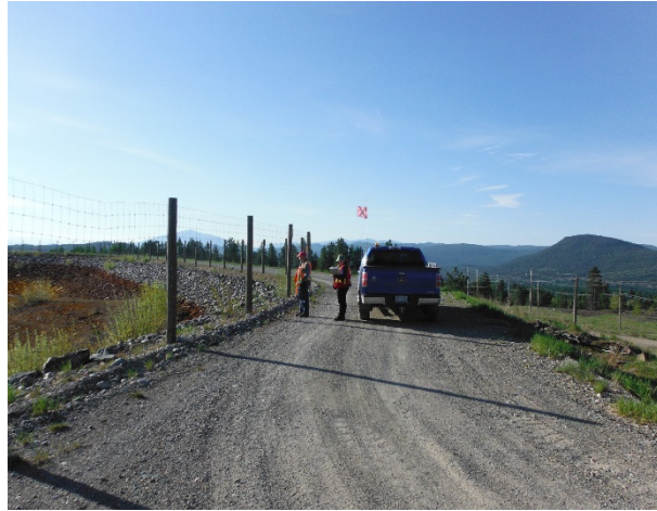
6.02: May 10, 2017 Crest of ARD South Dike
