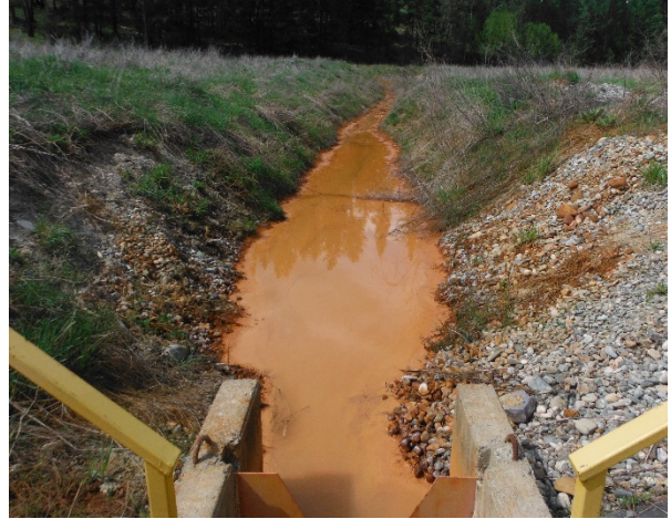
1.14: May 10, 2017 Weir #4 (Old Weir)
