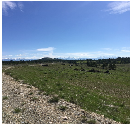
5.24: May 10, 2017 East Gypsum Dike crest
