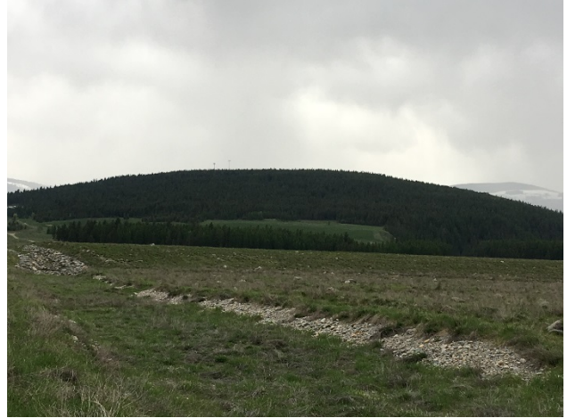
4.14: May 11, 2017 Drainage channel from Dike #1 to Emergency Spillway
